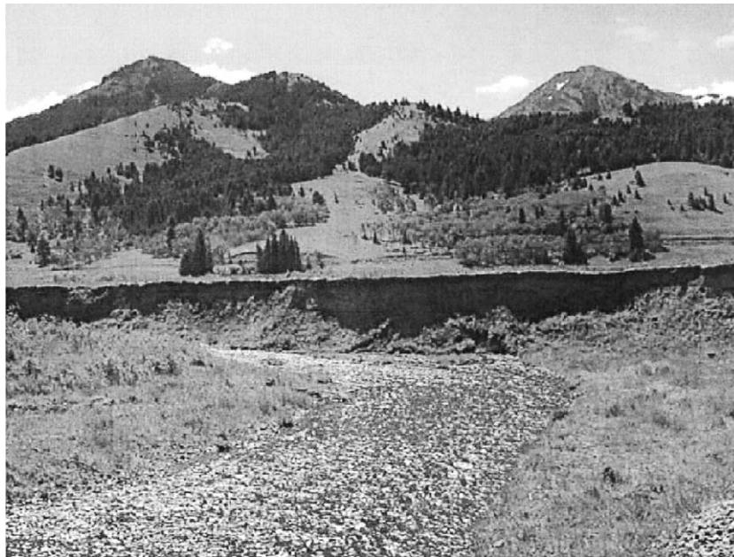
Fig. 3. Extensive right bank failure on Tom Miner Creek.
